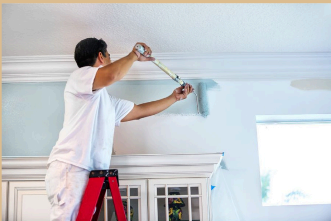
INTERIOR WALL PAINTING
